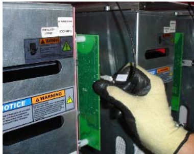
Figure 8-6: Fiber Optic Cable Removal/Installation
