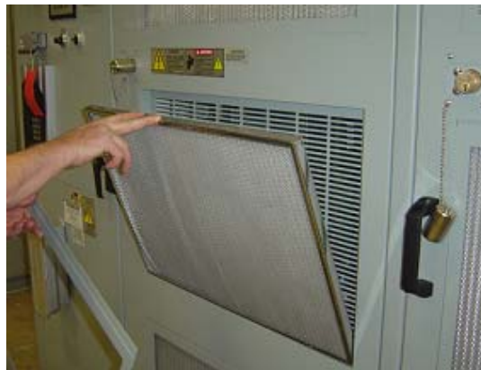
Figure 8-3: Filter Removal
