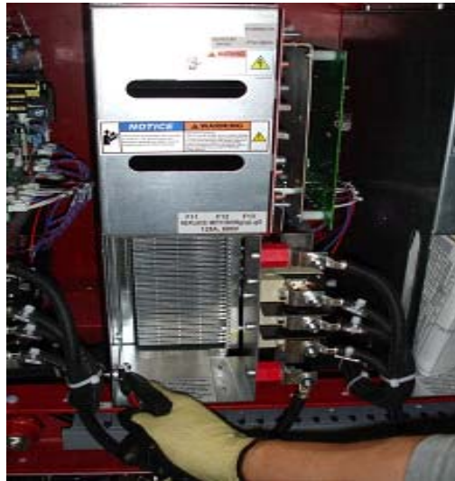
Figure 8-8: Bolt Removal
