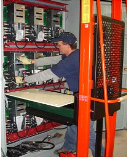
Figure 8-10: Sliding the Cell onto the Lifter
